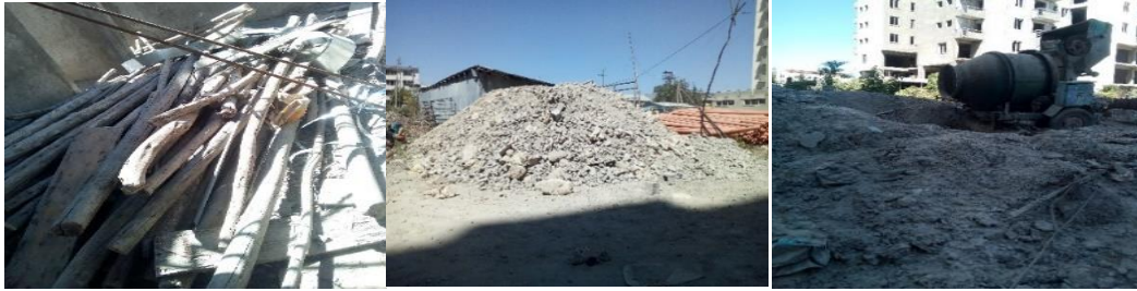
Figure-2 Wastes created on conventional construction system on condominium site. (Source: Tourist site condominium, Megenagna)
